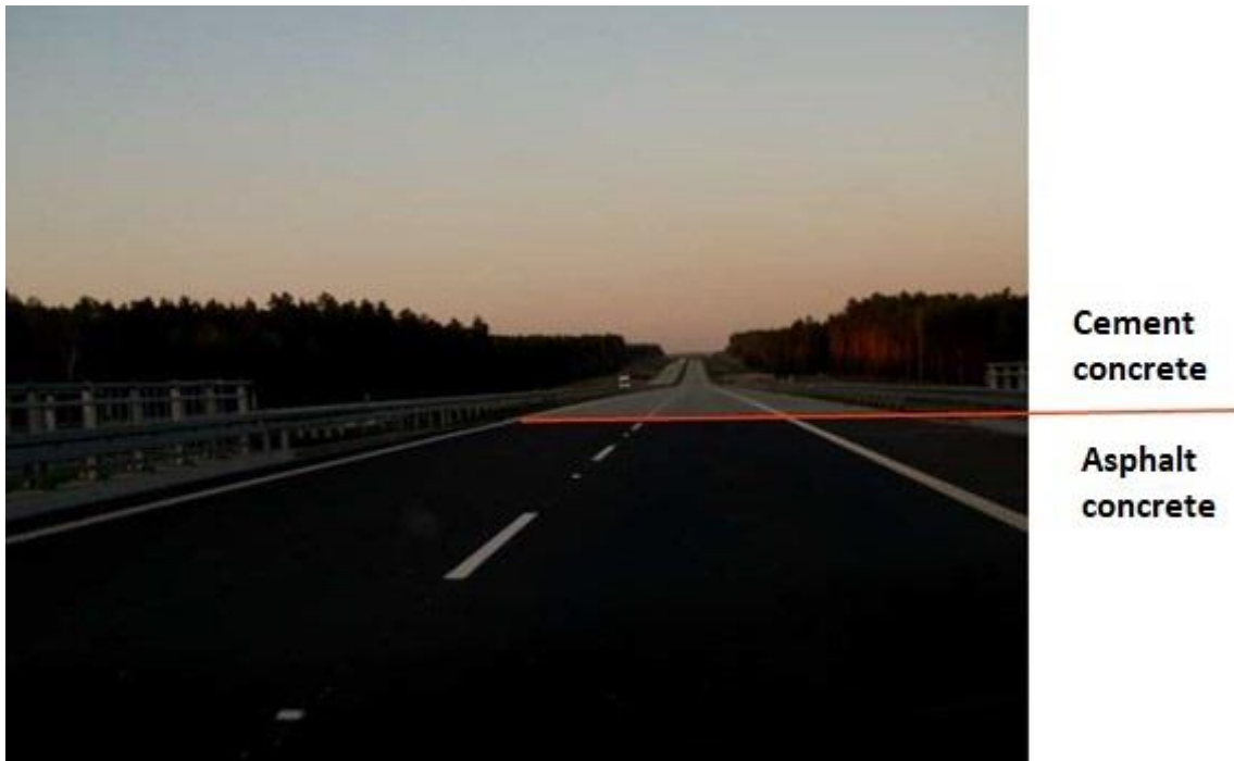
Figure 1. Comparison of the brightness (visibility) of a cement concrete and asphalt concrete road.
